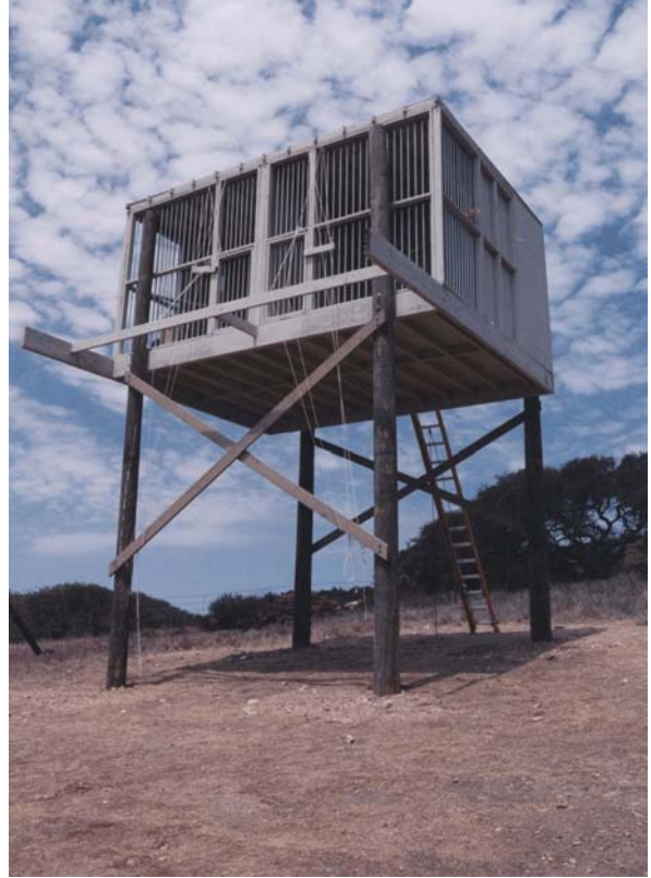
Figure 4. South hacking tower located on Santa Cruz Island, California.
